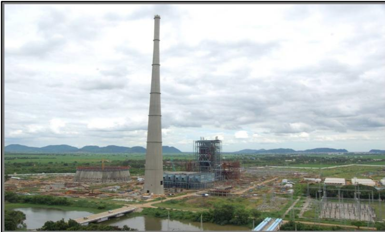
Vijayawada Thermal Power Station (Under Construction)
