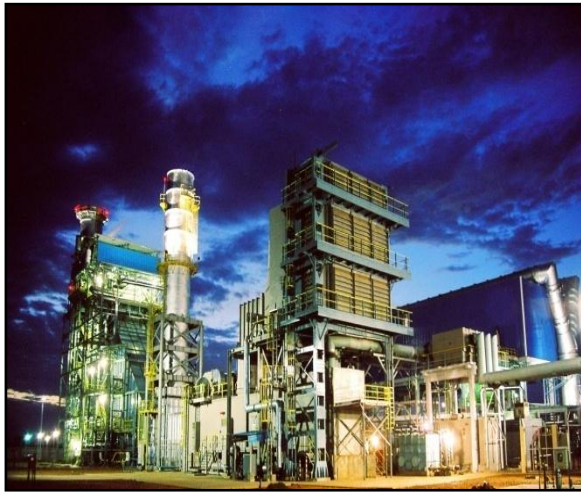
120 MW CCPP Aban Power, Karuppur, Tamil Nadu
