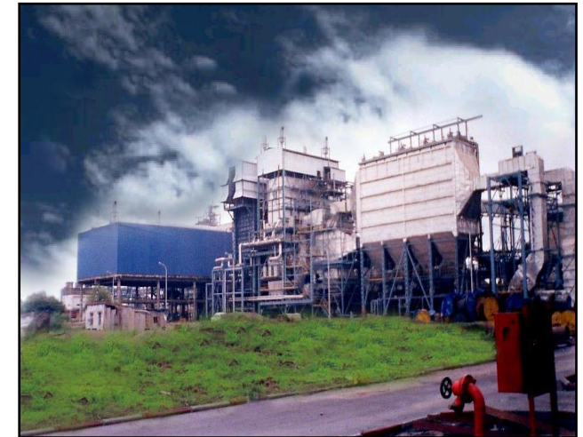
23 MW CPP Grasim Industries, Chittorgarh, Rajasthan
