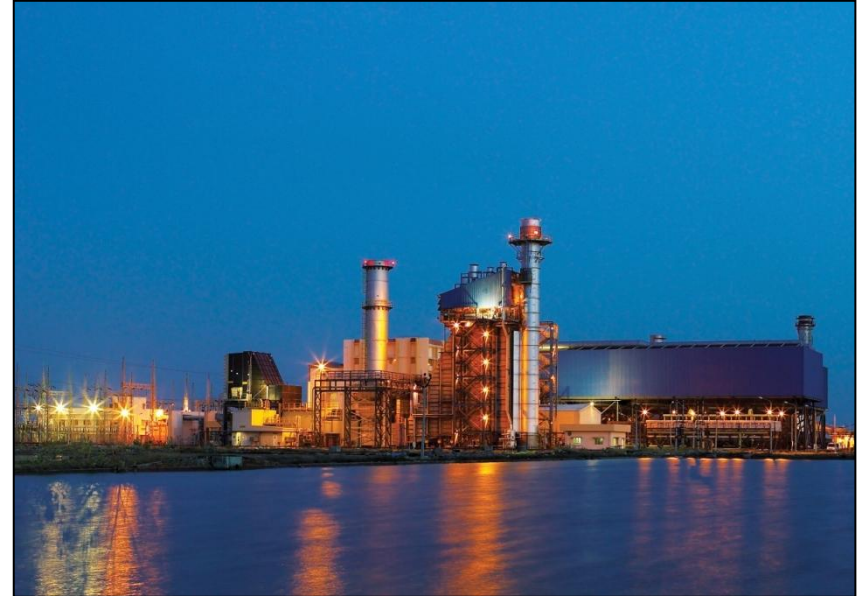
92.2 MW CCPP Valathur (Phase II), Tamil Nadu
