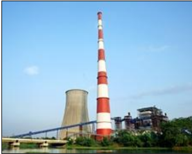
Vijayawada Thermal Power Station (Synchronized on 4 th Apr '09)
