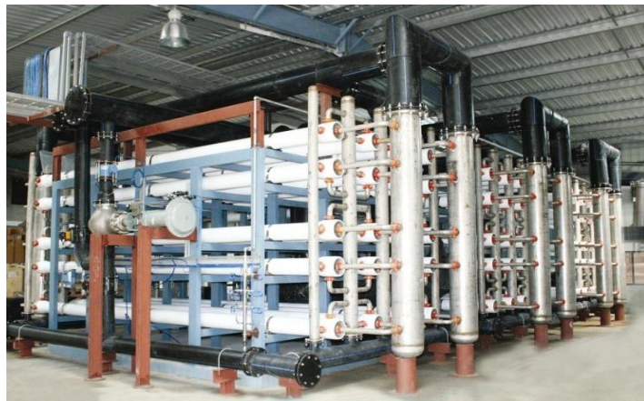
Effluent Recycling Plant – Tiruppur
