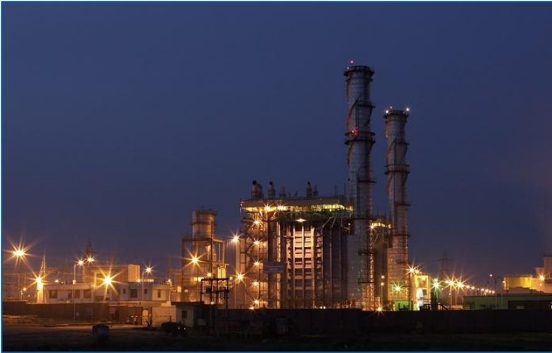
330 MW CCPP RRVUNL, Dholpur, Rajasthan
