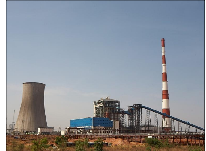
Kakatiya Thermal Power Station, Andhra Pradesh
