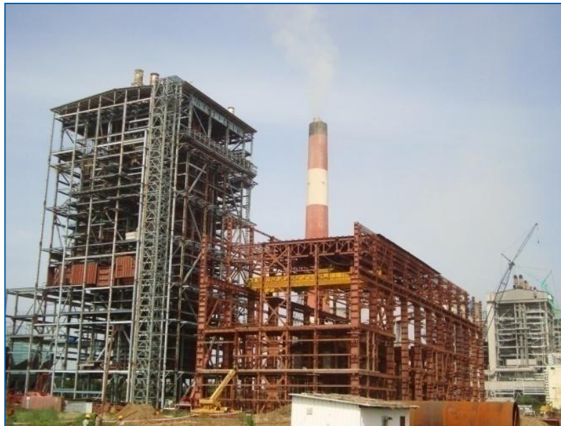
Kothagudem Thermal Power Station (Under Construction)
